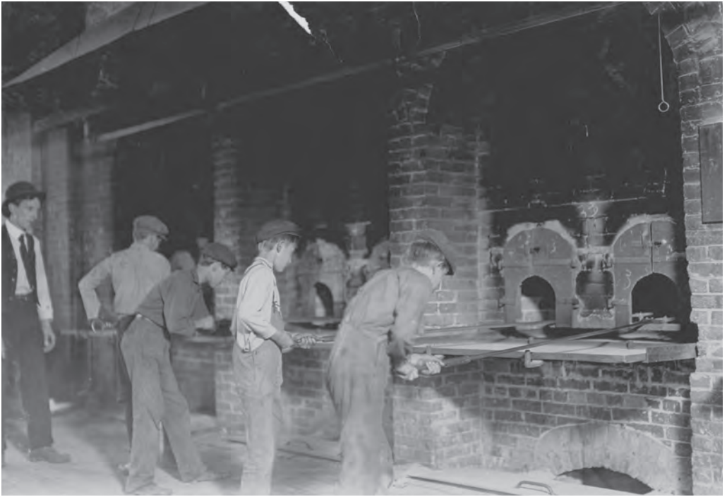
“Glass Works.” West Virginia, October 1908
