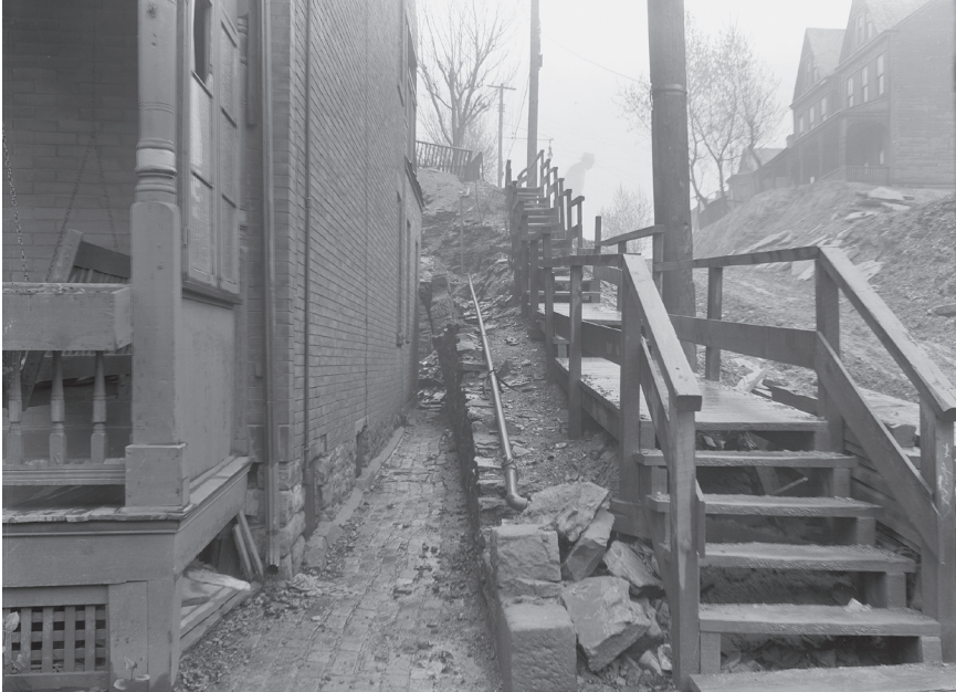
Fig. 1.2 Landslide damage, Shaler Street, June 17, 1920. Throughout its history Pittsburgh has suffered extensively from landslides (Pittsburgh City Photographer Collection, courtesy of the Archives Service Center, University of Pittsburgh).
