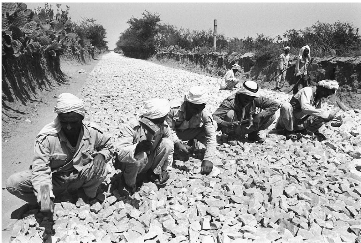
Figure 1.1. Local laborers employed by Israel's Public Works Department lay the foundation of a new road from Khan Yunis to the Jewish kibbutz Nirim, in the Negev, 1969. Moshe Milner, The National Photo Collection.
